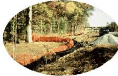
5. Erosion & Sediment Control
